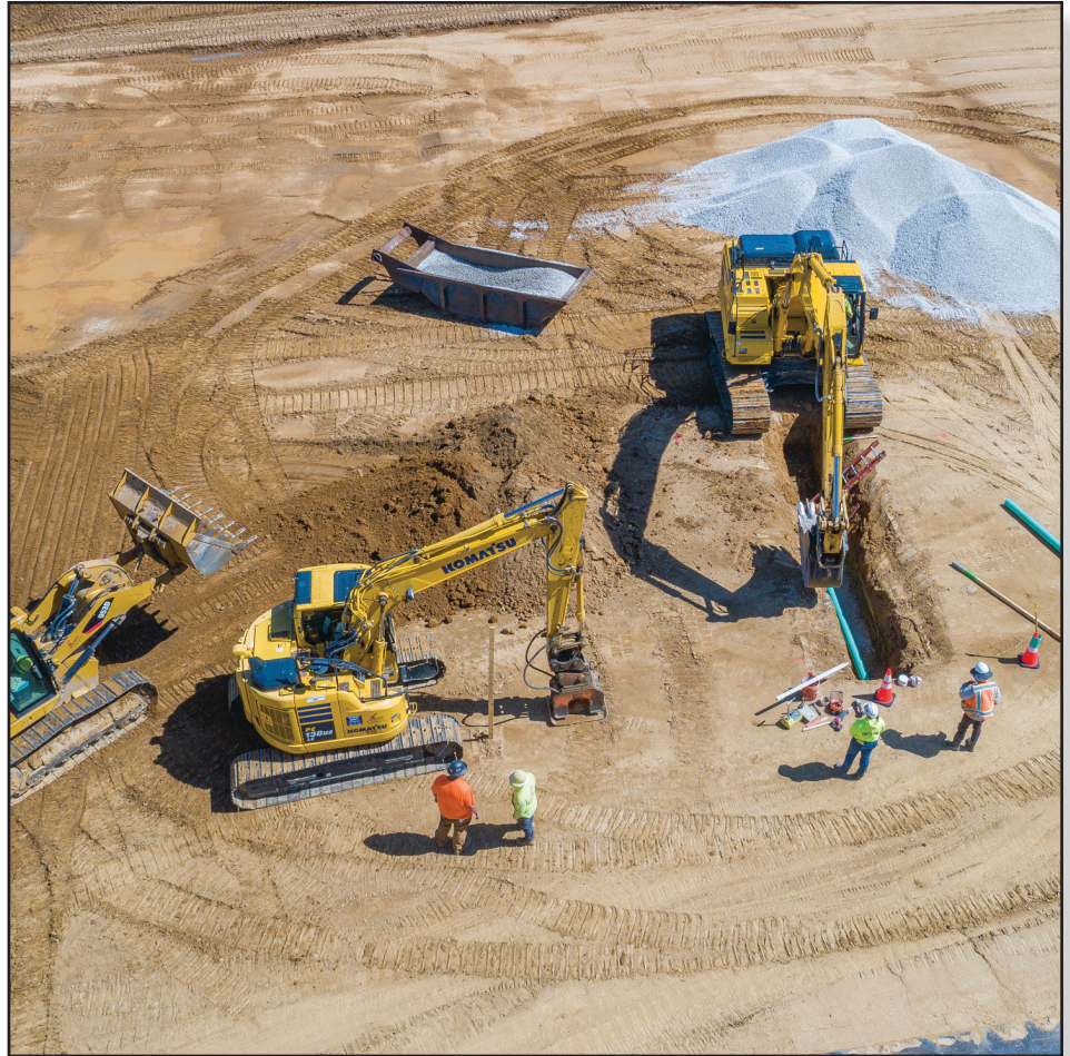
▲ At Honeybrook Estates, a Schlouch utility crew installs sanitary laterals for the 37 single-family lot subdivision.
