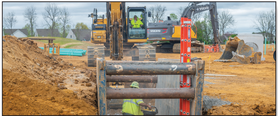
▲ At The Villages of Wolf's Run Phase 1, a Schlouch utility crew installs sanitary main for the 103-unit townhouse subdivision.
