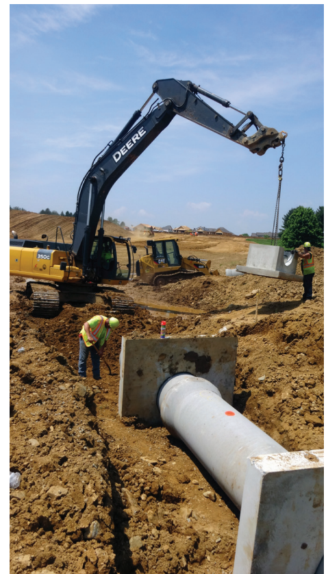
▲ Schlouch pipe crew installs storm water drainage pipe for 58 single family homes at the “Fields at Indian Creek Phase 3” site, located in Upper Milford Township and Emmaus Borough, Lehigh County, PA.
