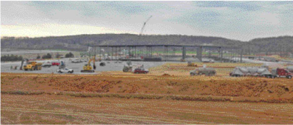
▲► *Nearing a fall completion, SI teams complete site grading, soil stabilization and pipework on a 52-acre site for Urban Outfitters (above and right).*
