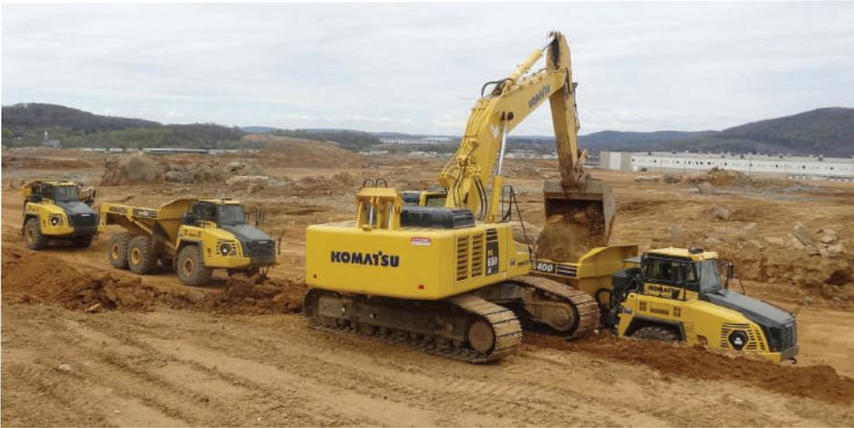
▲ Schlouch earthwork crew loads a train of large trucks as they prepare the pad for a 536,650 s.f. warehouse being constructed by Commerce Construction Co., L.P. in Bethlehem.
