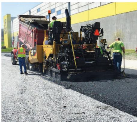
▲ Schlouch Incorporated is widening the access roads at Urban Outfitters Internet Fulfillment Center in Lancaster County. Here a crew installs porous paving materials as part of this project.
